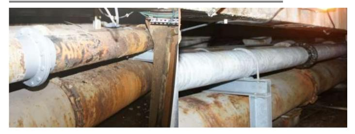
Resimac composite pipe repair products can be used to seal leaking pipework ranging from 1/2" (1.2cm) to 48" (121cm).
