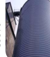
Grain silo required a 15 year + coating system to protect from further surface corrosion. The mechanically prepared surface was primed with 2 x coats of 506 Aluprime and top coated with 2 x coats of 508 UVPU
