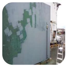
The external tank surfaces were mechanically abraded and primed using Resichem 501 CRSG, once cured a single coat of 508 UVPU was applied to give a UV stable finish to the tank surface
