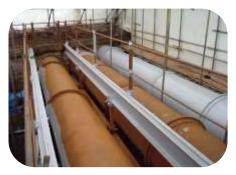
External pipe surfaces at a waste water treatment plant had become badly corroded. The surfaces of the pipes were mechanically abraded and protected with 2 x coats of 506 Aluprime
