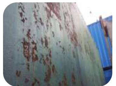
Diesel storage tank at a UK marina was badly corroded due to the corrosive environment. The external tank surfaces were mechanically abraded and protected using Resichem 501 CRSG.
