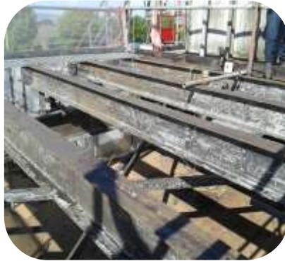
Structural steel underneath a water tank abrasive blast cleaned and coated with Resichem 501 CRSG
