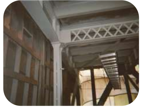
Structural steel underneath a water tank abrasive blast cleaned and coated with Resichem 501 CRSG
