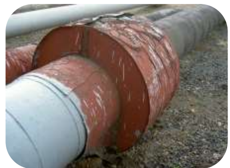
Badly corroded pipe surfaces were hydro-blasted at a European refinery and coated with 2 x coats of Resichem 501 CRSG to give long term protection against CUI
