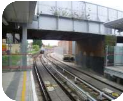
Bridge over UK rail line mechanically abraded and coated with 2 x coats of Resichem 501CRSG. Once cured Resichem 508 UVPU was applied to give a UV resistant finish
