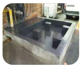
Chemical containment area and sump rebuilt with 577 Chem Screed and overcoated with Resichem 511 UCEN
