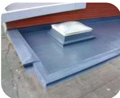
Factory roof protected using the 557 Polyroof EC & 558 Polyroof UV system
