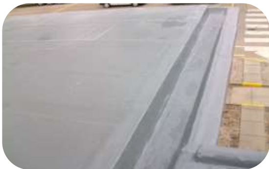
Factory roof resurfaced using 552 CSM Membrane and 550 WR Membrane top coat
