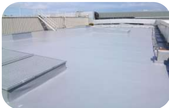
Factory roof resurfaced using 552 CSM Membrane and 550 WR Membrane top coat
