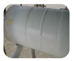
Resichem 530 HA100 applied by brush to pipe field joints, while the coating was still wet Polypropylene was flame sprayed onto the surface of the Resichem 530 HA100.
