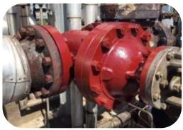
As part of the site improvement plan over 300 valves, pumps and spools were coated Resichem 530 HA100. The coating was applied to surfaces operating at  $150^{\circ}$  C. Surface preparation was high pressure water jetting at 1000 psi to clean off any surface contaminants and the coating was applied at 300 microns per coat.
