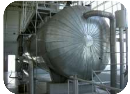
De-mineralised water tank operating at 100-110°C abrasive blast cleaned and lined using 206 Ceramic HTA
