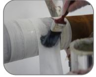
Once the entire length of pipe has been wrapped apply mixed resin to the pipe surface, wrap the tape 3 times around the pipe to terminate the repair
