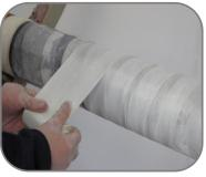
After the pipe wrap has been terminated, apply another layer 301 Epoxy Resin & Hardener at 500 microns WFT and repeat the glass tape wrapping
