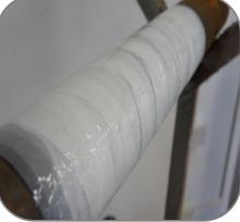
The completed system will range from 2-5mm dry film thickness depending how much 302 Epoxy Repair Cement has been applied.
