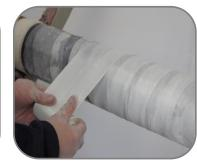
After the 2<sup>nd</sup> wrap of glass tape has been terminated. Apply 301 Epoxy Resin & Hardener at 500 microns WFT and repeat the glass tape wrapping process for a 3<sup>rd</sup> and final time
