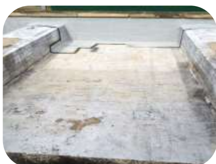
Concrete surface on a chemical containment area was mechanically abraded and sealed with Resichem 503 SPEP prior to being over coated with Resichem 501 CRSG
