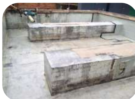
Concrete surface on a chemical containment area was mechanically abraded and sealed with Resichem 503 SPEP prior to being over coated with Resichem 501 CRSG
