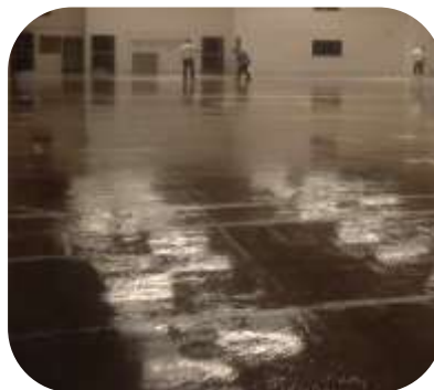
Concrete surface on a chemical containment area was mechanically abraded and sealed with Resichem 503 SPEP prior to being over coated with Resichem 501 CRSG
