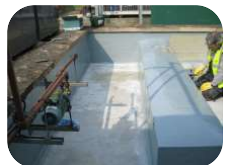
Concrete surface on a chemical containment area was mechanically abraded and sealed with Resichem 503 SPEP prior to being over coated with Resichem 501 CRSG
