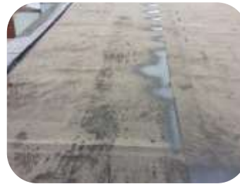
Mineral felt roof with leaking joints sealed with 2 x coats of 554 RB Membrane
