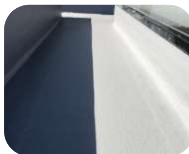
New roof construction waterproofed with 554 RB membrane and glass fibre matting
