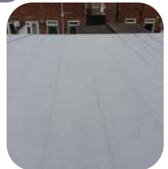
Mineral felt roof with leaking joints sealed with 2 x coats of 554 RB Membrane
