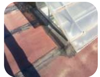
Leaking seams on a mineral felt roof sealed using 551 ER Membrane
