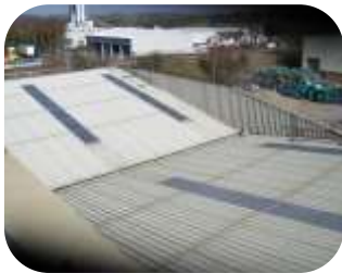
Over 600 linear meters of GRP valley gutter sealed with 551 ER Membrane
