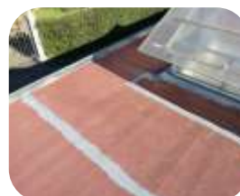
Leaking seams on a mineral felt roof sealed using 551 ER Membrane
