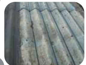
2000m 2 corrugated metal roof coated with 2 x coats of 550 WR Membrane
