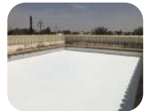
3000m 2 flat concrete roof coated with 2 x coats of 550 WR Membrane
